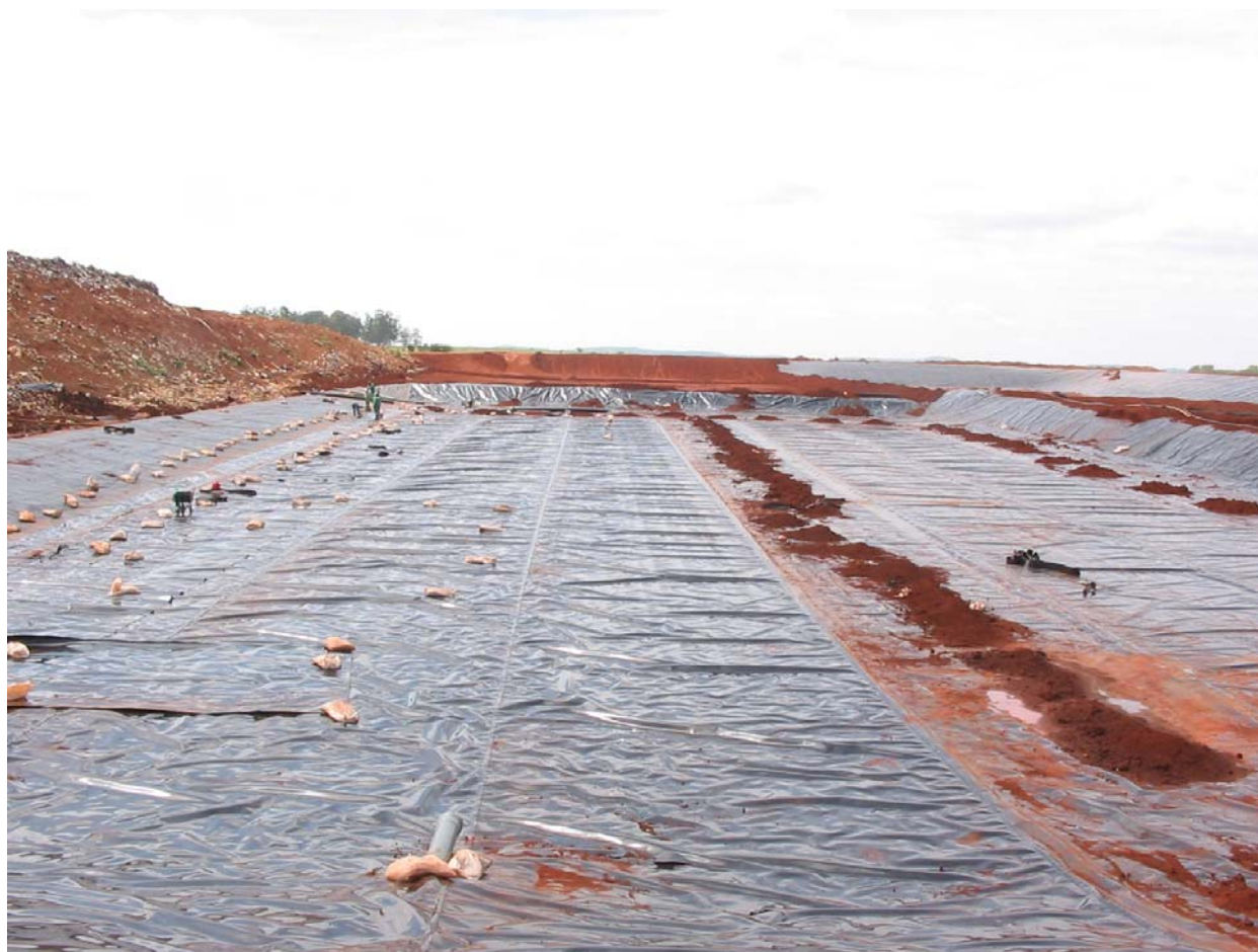
Figure 4: Geomembrane installation on cell 3
