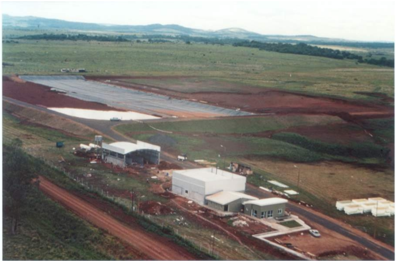
Figure 2 Aerial View of the Fachinal Sanitary landfill
